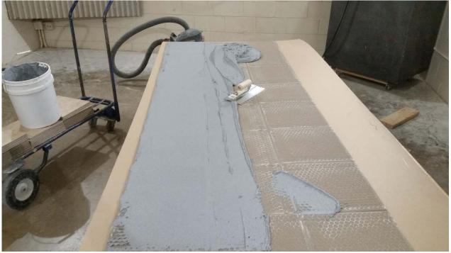
Figure 2 – Pretreatment of tiles with smooth mortar layer
